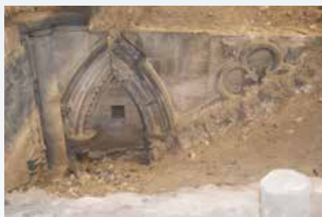
11. The remains of the eastern lantern still in situ above the vault over the high altar. The original intention to build a lantern tower in this area was abandoned when it fell off in the early 13th century.
